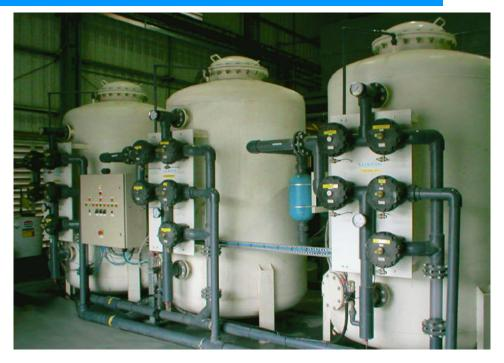
Lubron's range of pressure filter systems is readily configured for removing both particulates and various dissolved species in effluent, ground, process and surface waters.
