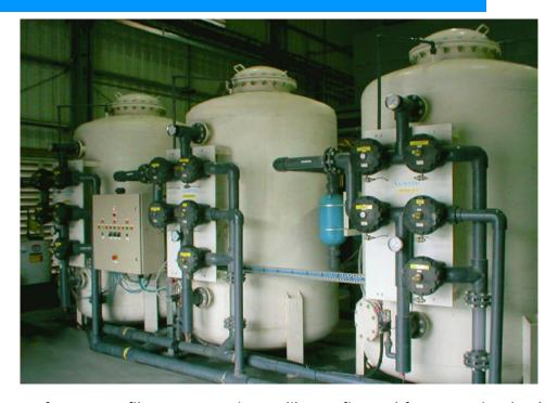
Lubron's range of pressure filter systems is readily configured for removing both particulates and various dissolved species in effluent, ground, process and surface waters.
