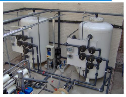
Lubron's range of pressure filter systems is readily configured for removing both particulates and various dissolved species in effluent, ground, process and surface waters.
